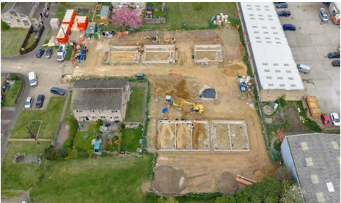
Wellington Way - On Site Aerial Progress Photo - 30 th April 2026.
